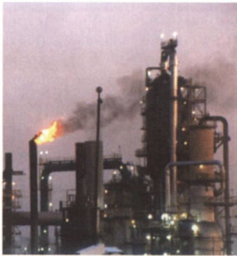
Figure 61 Flames coming out of stacks of fired heaters after tube ruptures.
