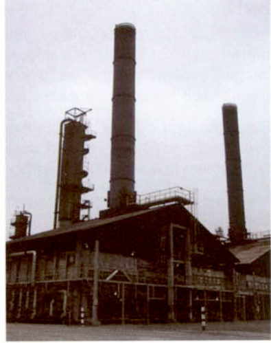
Figure 5a Multiple box type furnaces.
