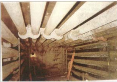
New roof hangers.
